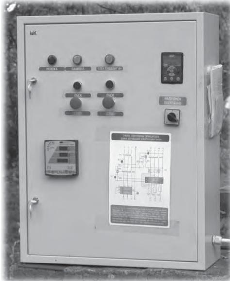
FIGURE 5. Automated system based on the motor control unit Danfoss Micro Drive
